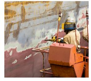
Surface cleanliness is the prime requirement for good, holiday-free coating practice. METgrain's mix of hard, irregular-shaped metallic particles maximize blast cleaning efficiency for removing paint, rust, and mill scale. The result is a cleaner surface, with a high-speed cleaning at a lower cost.
